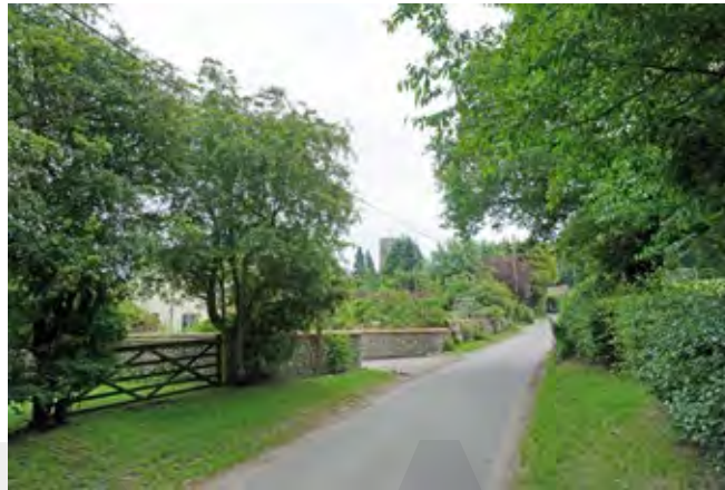
Showing the sensitive transition to the newly built red brick and flint wall beside the historic wall on properties east of Brinton Road
