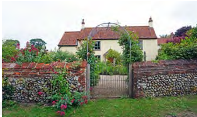
Rose Cottage, rendered with red clay pantile roof, east of Brinton Road
