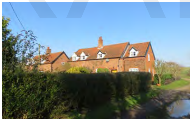
Beck Cottages are parallel with Hunworth Road accessed via Barbers Lane
