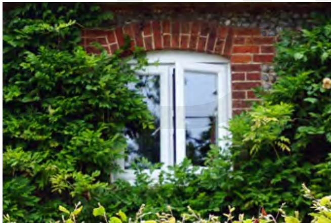
Inappropriate uPVC windows
