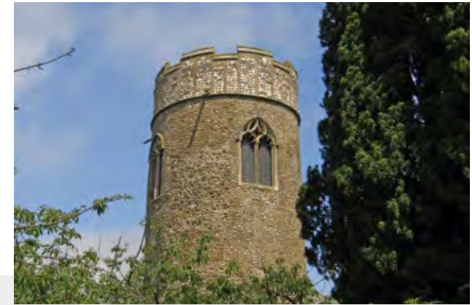
View of knapped flint trefoil pattern on upper part of church tower
