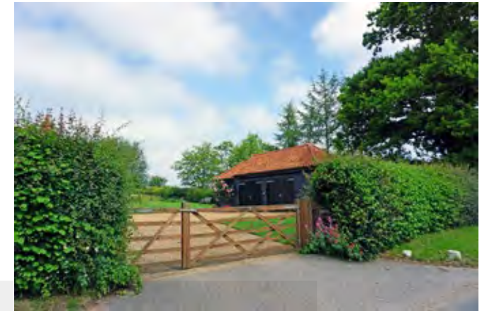
View of modern built garage with use of traditional materials of weatherboarding and red clay pantiles
