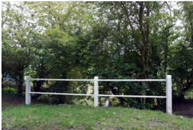
Typical fence on the bridges over the becks
