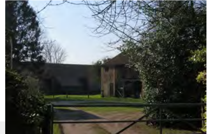
The two Grade II listed barns at Kendles Farm
