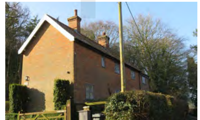
Coronation Cottage is a rare mid-twentieth century addition to Study in red brick
